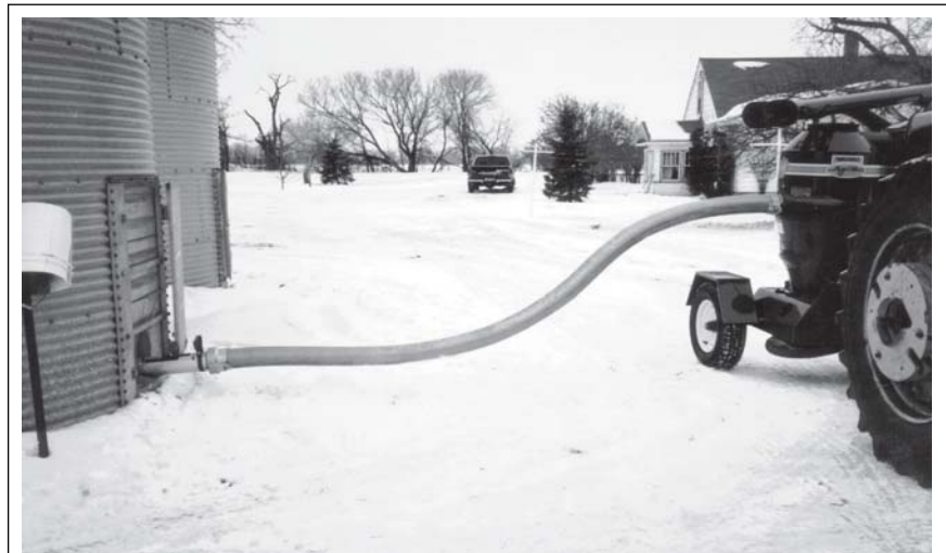
Fig. 12 FLEX TUBE INSTALLATION
