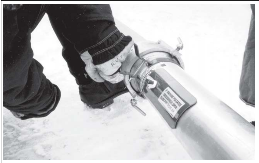
Fig. 11 INTAKE INSTALLATION
